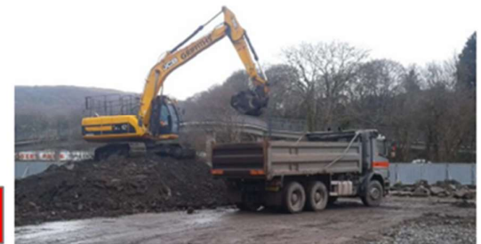
Right: Arisings being saved from land fill to be put to good use elsewhere
