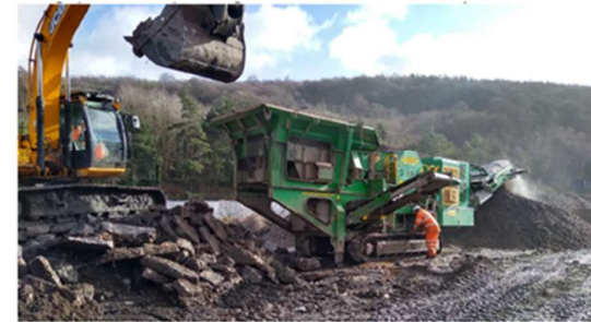
Above: Crusher in use producing 6F2 from concrete slab
